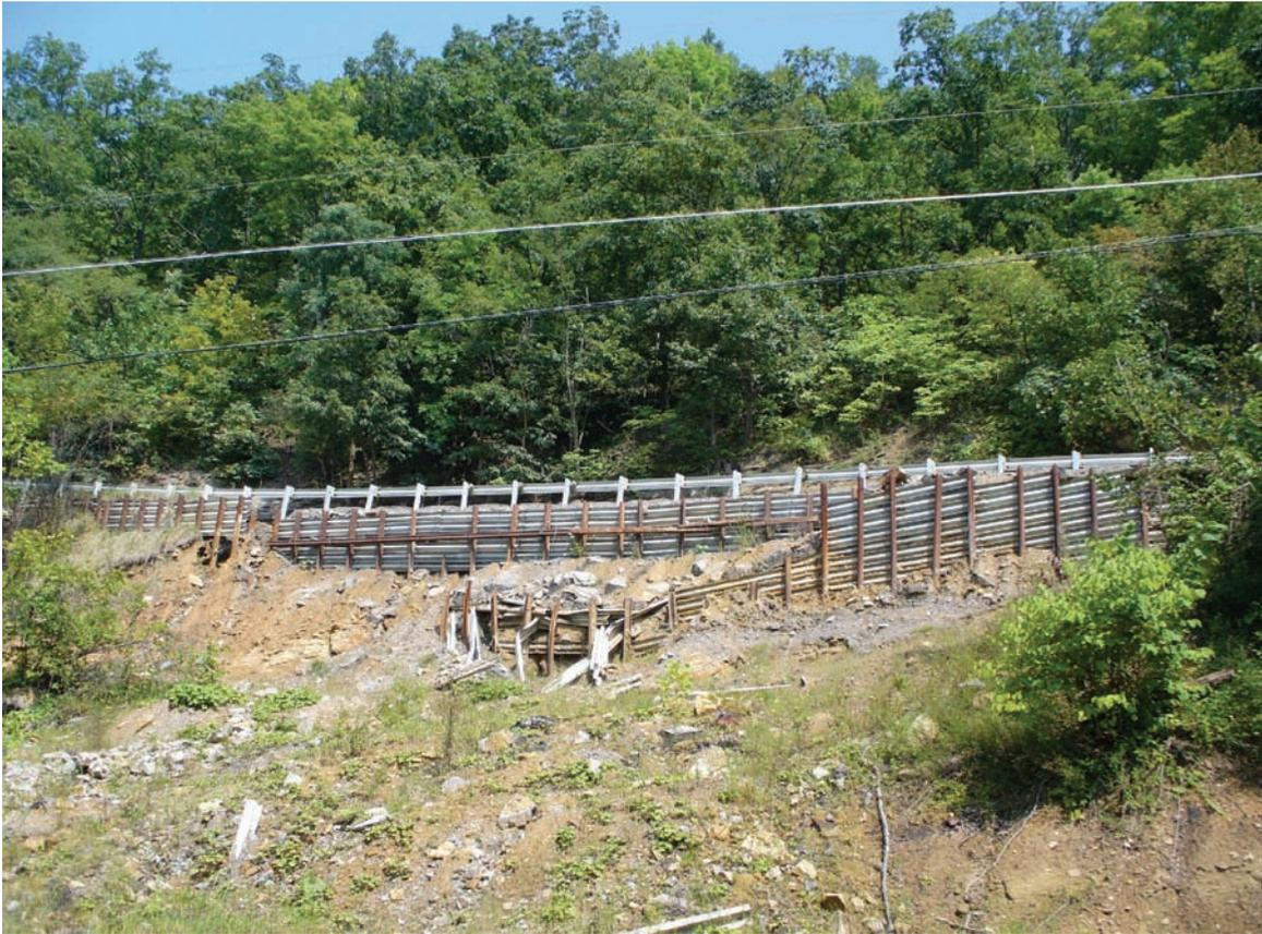
**Mountainous topography can make road construction difficult. Rights-of-way are often extremely steep, and subject to landslides, as in this case in northern Pike County on Ky. 881 built on the Four Corners Formation. Photo by Bart Davidson, Kentucky Geological Survey.**
